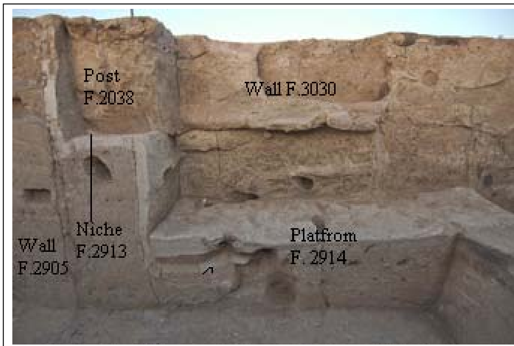
Figure 26: East wall and features of Space 67.
