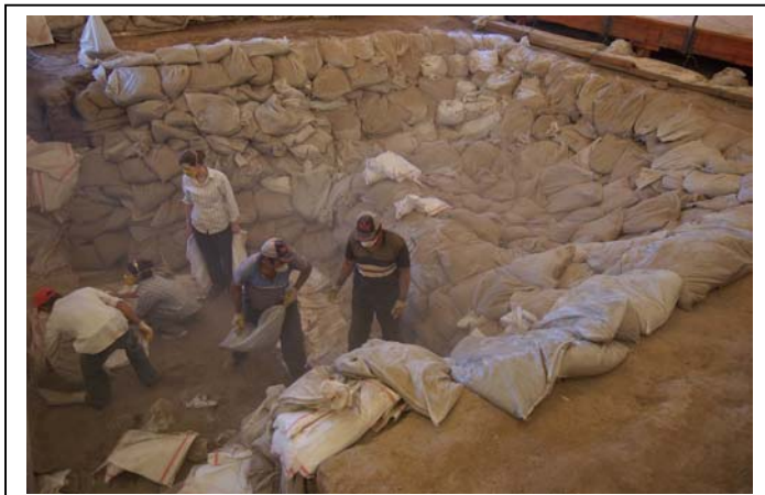
Figure 177: Building 5 during reburial with perlite and sand bags
