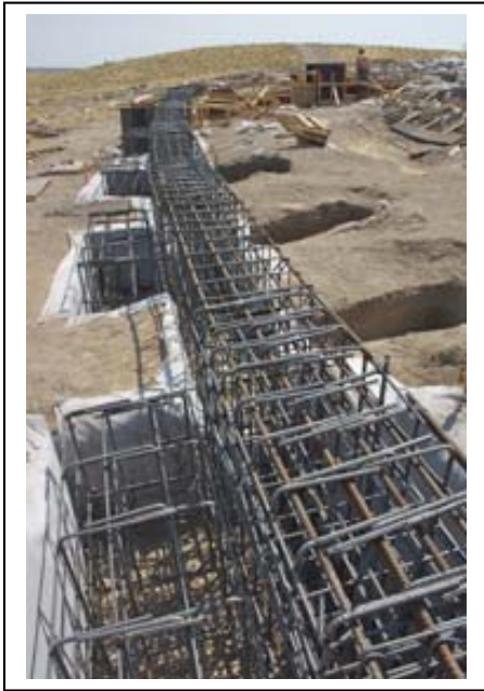
Figure 11: The Foundation Trenches were lined with geotextile with a basal layer of gravel before the steel reinforcement was fashioned in situ.
