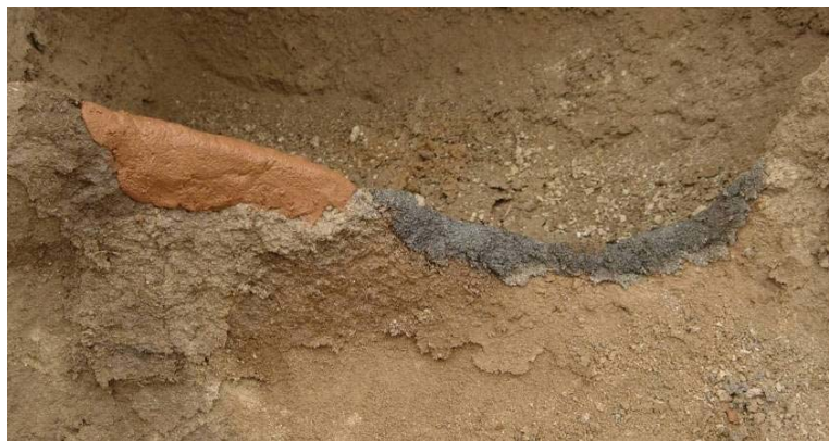
Figure 129: Clay mixed with 50% Primal AC-33 and a mortar applied to a test area of the bins of Building 5. Photo Graeme McArthur
