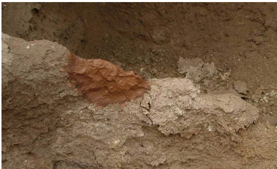
Figure 127: clay mixed with 25% Primal AC-33 applied to the Building 5 bins. Photo Graeme McArthur
